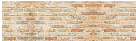
M24 Brick wall
